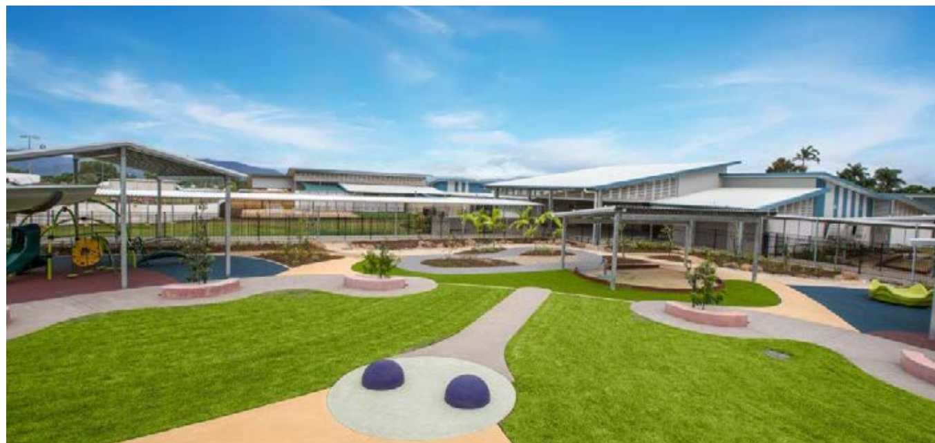
Urban Design at the newly built Cairns Special School, Cairns QLD
