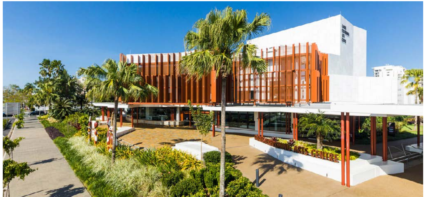
Cairns Performing Arts Centre, Cairns, QLD - Designed by LA3
