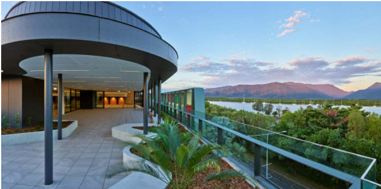
Cairns Convention Centre, Cairns , QLD - Designed by LA3
